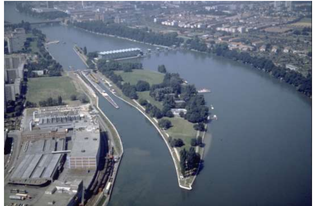
Birsfelden run-of-river power plant on Rhine River
